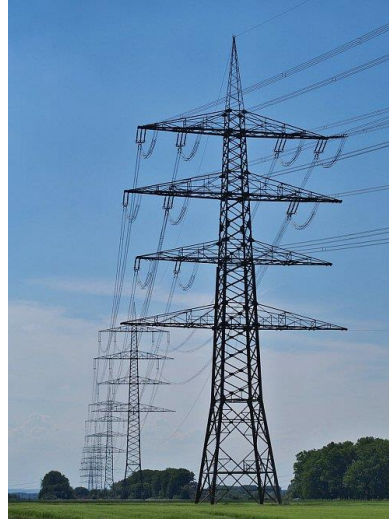
Figure 2.2: Transmission tower of a 380-kV line
