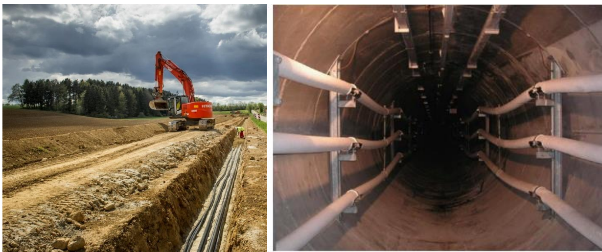
Figure 4.1: Laying of underground cables
