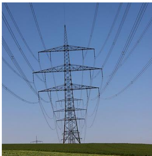
Figure 3.1: Upgrade of a 220-kV line to a 380-kV line
